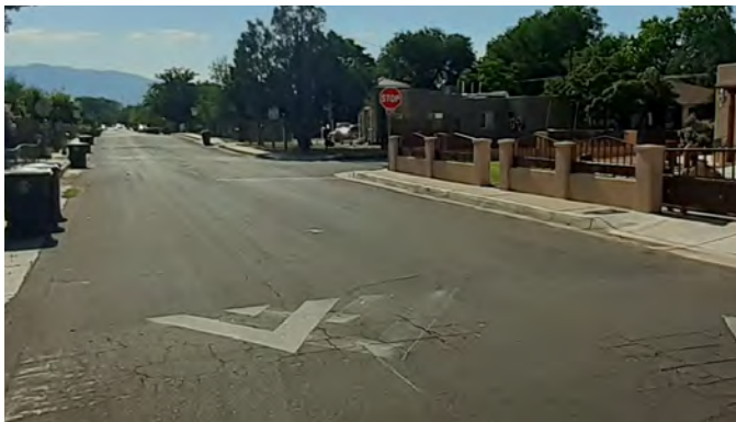
Residential Street with Speed Humps (Delamar Ave.)
