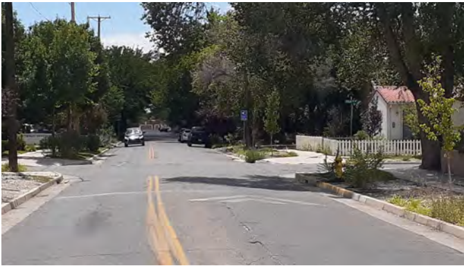
Collector Street with Speed Humps (12th St. South of Lomas)
