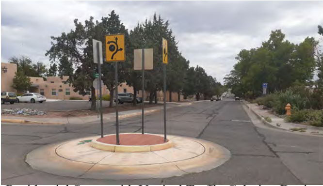
Residential Street with Vertical Traffic Calming Device (Dartmouth and Roma)
